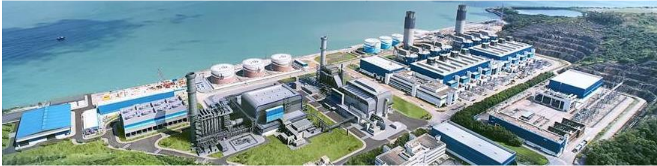
Black Point Power Station – gas fired combined cycle gas turbines
