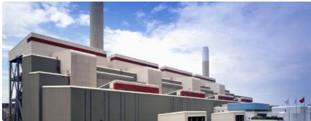
Castle Peak Power Station – coal fired steam turbines
