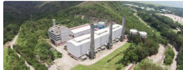
Penny's Bay Power Station – oil fired open cycle gas turbines
